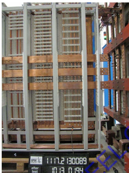
Photo 7: Test object after the verification of short-circuit withstand strength of busbar F1 in panel 2
