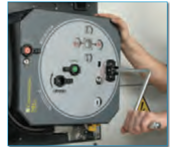
6 Lock the air rotary isolator in "open" position
