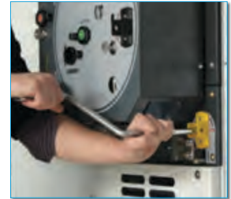
3 Open the earthing switch
