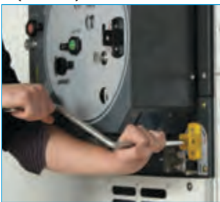
9 Close the earthing switch
